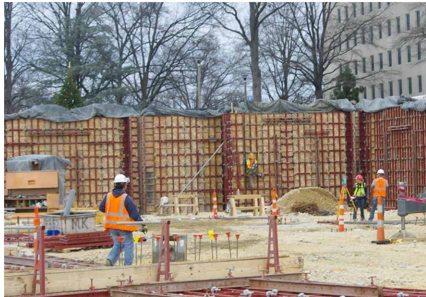
The Sym-Clamp allows crews to quickly assemble or reconfigure gangs.
