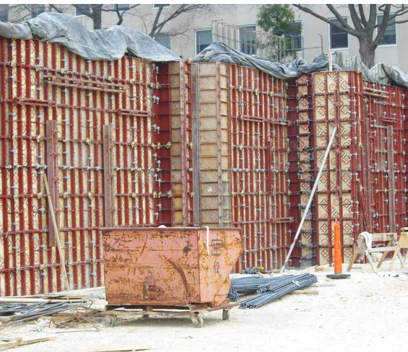
Sym-Ply can be used with Steel-Ply® forms to make details, such as odd dimensions at corners, simple and productive.
