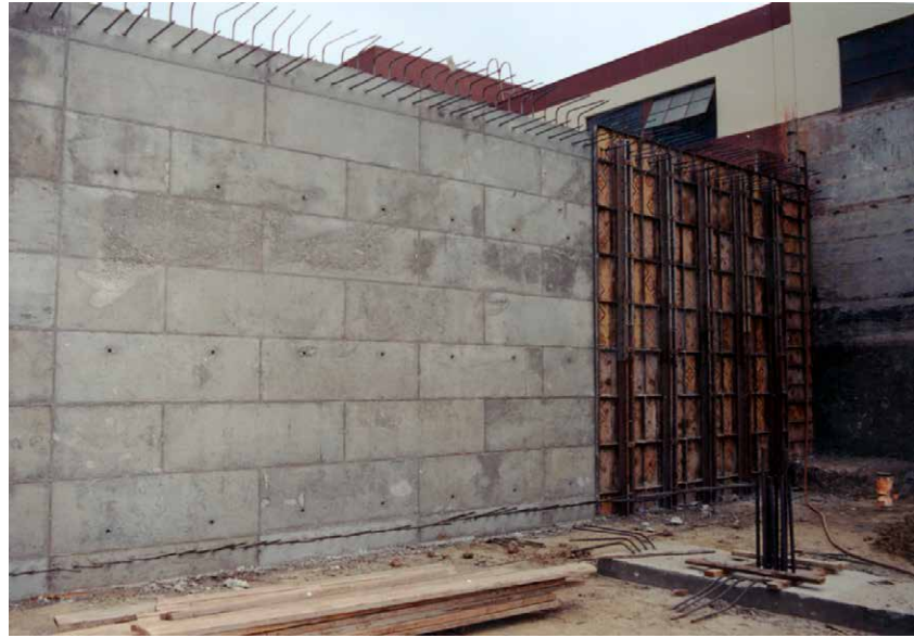
The widely spaced tie holes allowed with horizontal Steel-Ply reduces material and labor costs associated with ties and tie hole patching.
